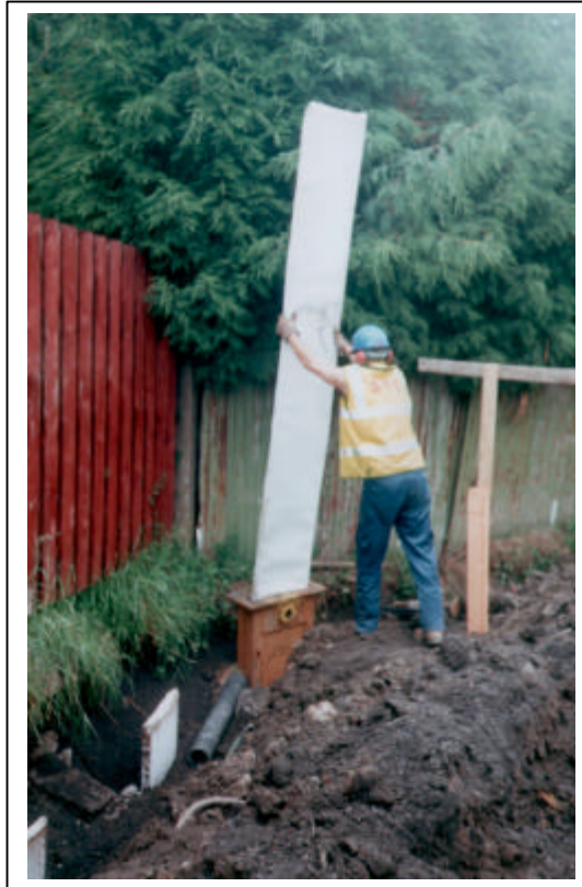
Figure 5 Inserting geocomposite vents into ground
