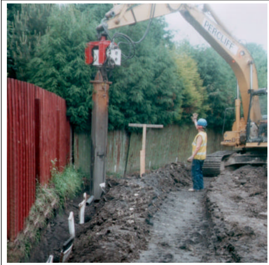
Figure 4 vibrating mandrill into ground
